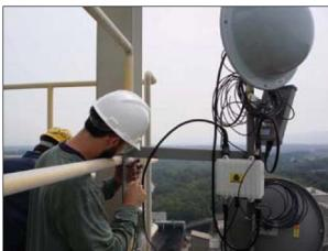
Figure 2 Installation of sector antennas and wireless router.
