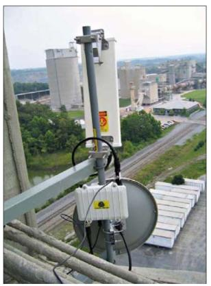
Figure 4 2.4 GHz sector and 5.8 GHz backhaul dish antenna
